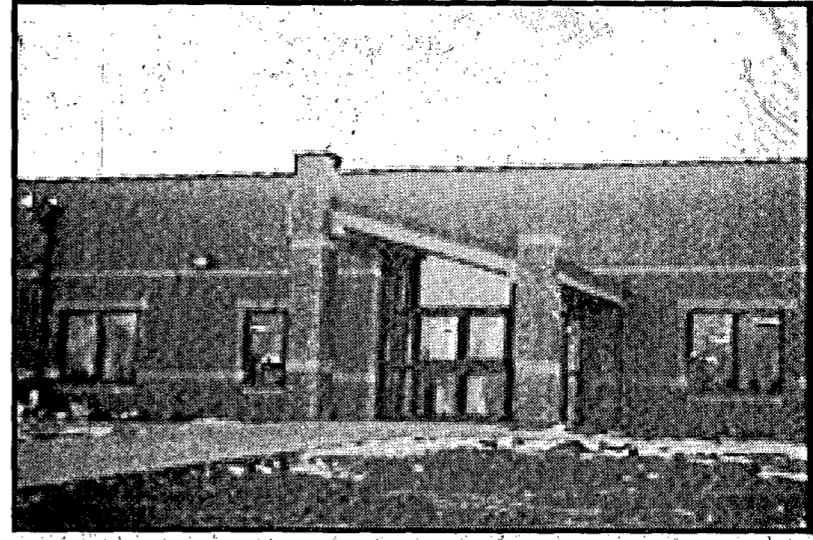
This is the new classrooms which have been constructed in Allen. Those attending Sunday's open house will be able to tour the facility.
